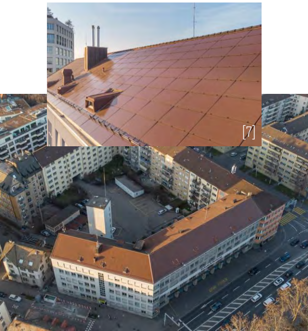
3S Swiss Solar Solutions AG Terracotta foil BIPV modules, Zurich (CH)
