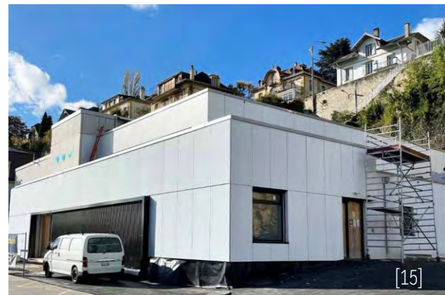
Solaxess 1 st generation of white foil, BIPV façade (CH)
