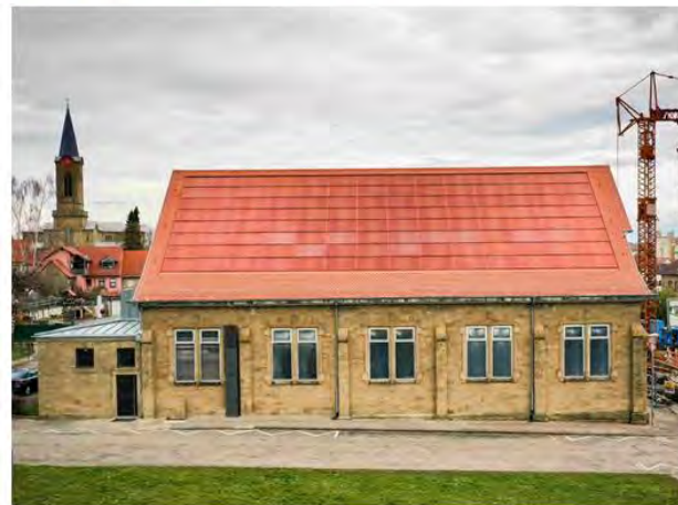
A building in Eppingen, Germany, with a red roof-integrated PV system
